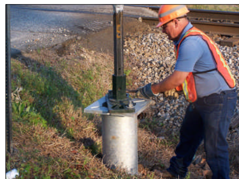
Completion of Installation
