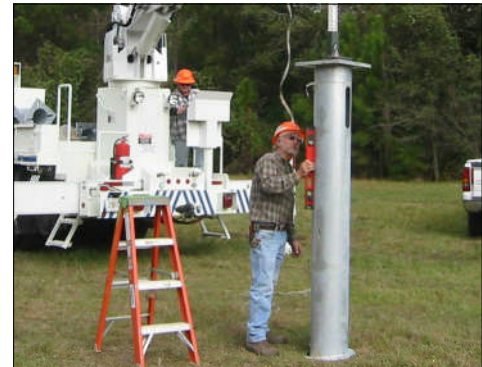
Checking Plumb
